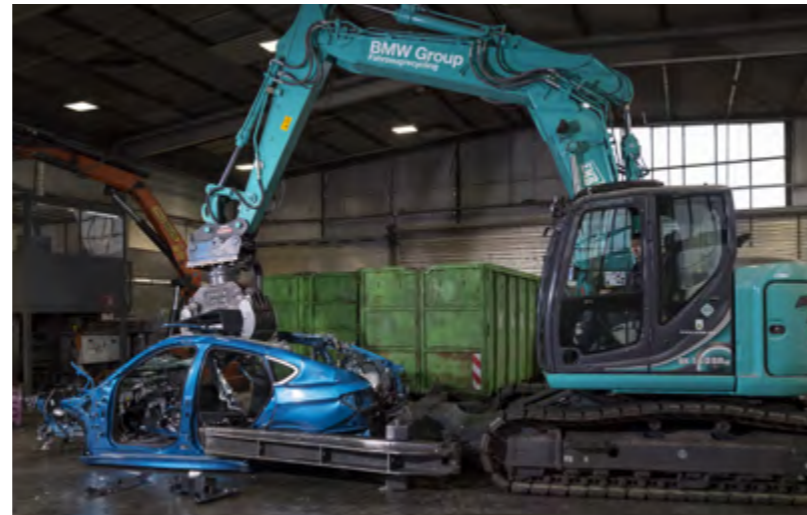
From the body to the cable harness: old vehicles are scrapped at the recycling and disposal plant.
