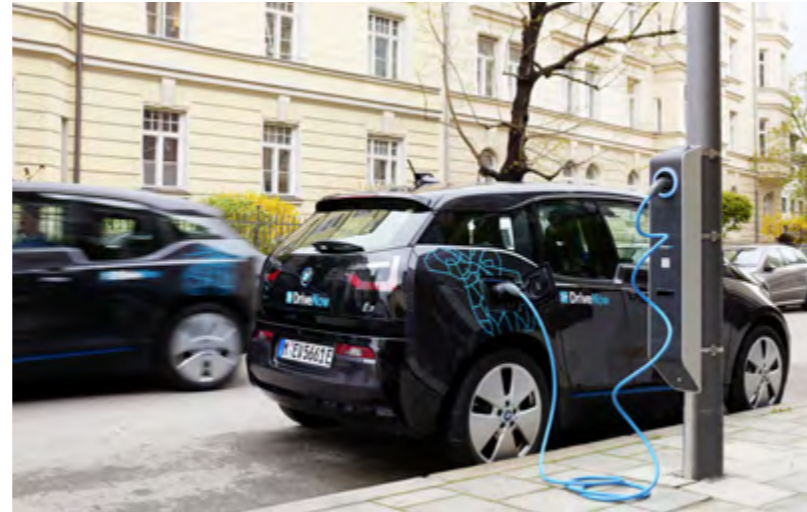
Charging at street lights: with Light & Charge, urban electricity sources become charging stations.
